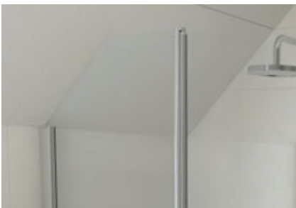
■ Bevel cut on fixed element
